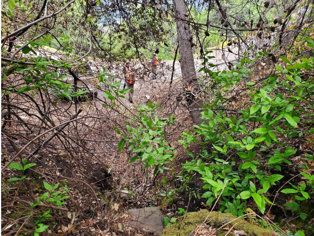
Photo 39. Site 147: View of the stream crossing from the left cutbank. The current CMP is near flat and long lengths of ditch flow utilize this crossing. The new CMP will be 36 inches in diameter and will be set at the natural stream grade.
