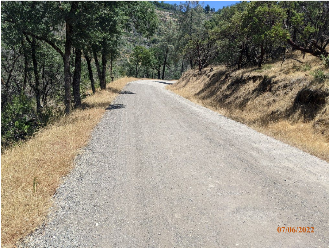
Photo 23. Site 134 : View looking uproad from OBR. RD#19.
