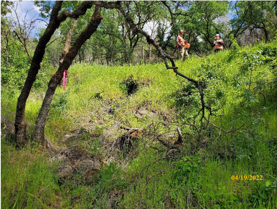
Photo 19. Site 131: View looking upstream at the current CMP outlet and outboard fillslope. A new 30-inch CMP will be placed at the base of fill.
