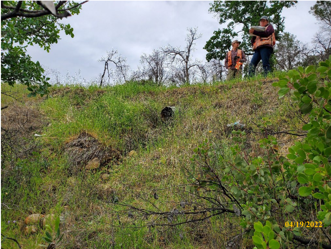
Photo 7. Site 124: View looking upstream at the current CMP outlet and outboard fillslope. A new 24-inch CMP will be placed at the base of the fill.
