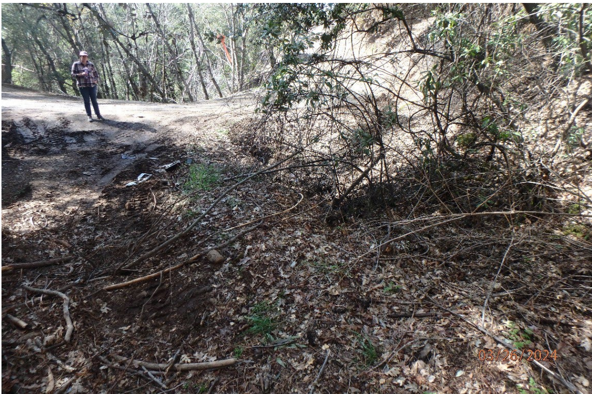
Photo 44. Site 149: View looking downstream towards the stream crossing culvert inlet area.
